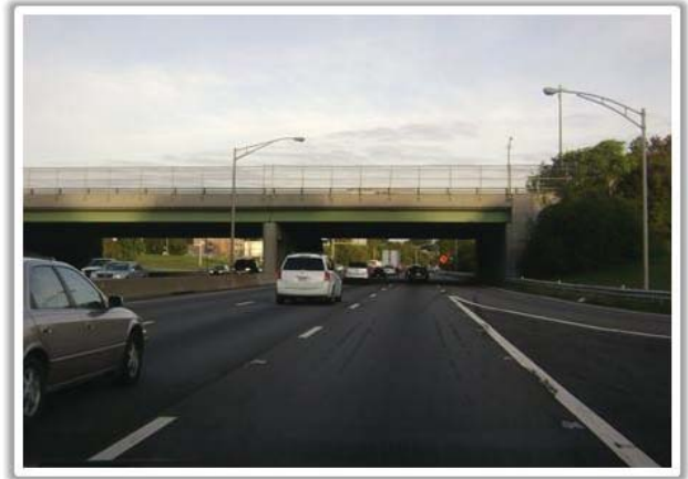
Photograph 5: Northbound I-95/I-64 Approaching the Belvidere Street On-Ramp
