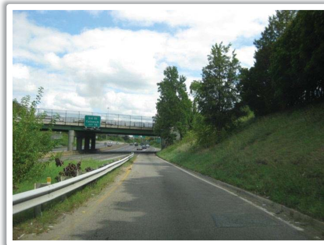
Photograph 4: Looking East from Merge Point of Upstream On-Ramps from Belvidere Street
