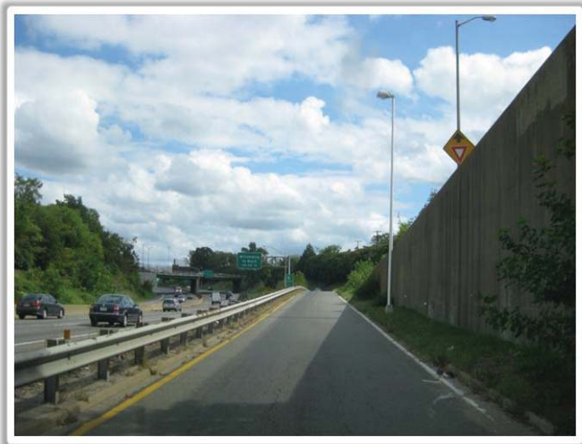
Photograph 2: Looking East from Collector-Distributor Road from Belvidere Street Loop On-Ramp
