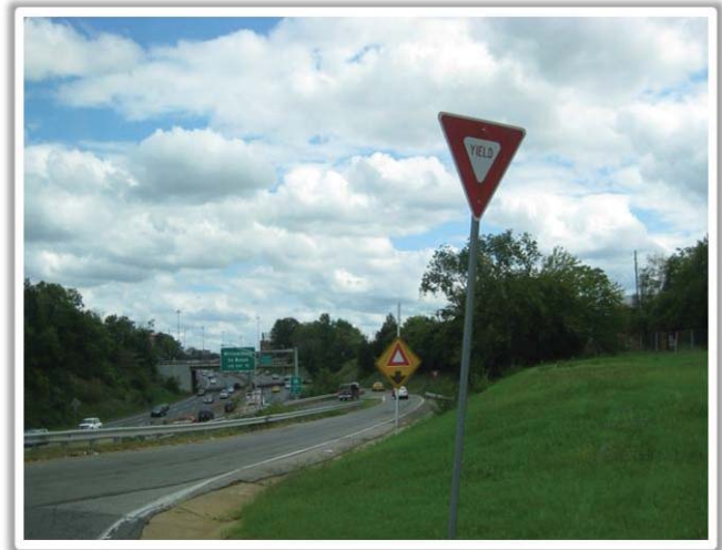
Photograph 3: Looking East from Slip Ramp from Leigh Street
